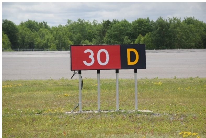
Figure 14 - Runway-Taxiway Intersection Mandatory Instruction Sign Located at a Runway Threshold
