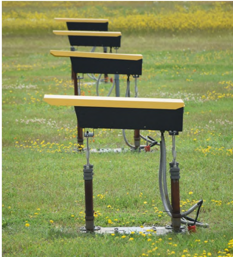
Figure 434 - Precision Approach Path Indicator (PAPI) Side View
