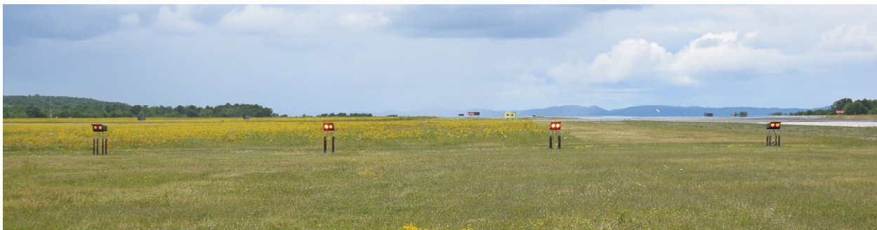
Figure 423 - Precision Approach Path Indicator (PAPI) Front View
