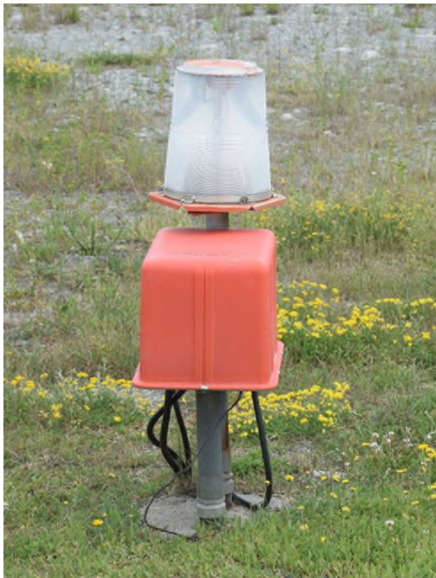
Figure 456 - Omni-Directional Approach Light (ODAL) Unit
