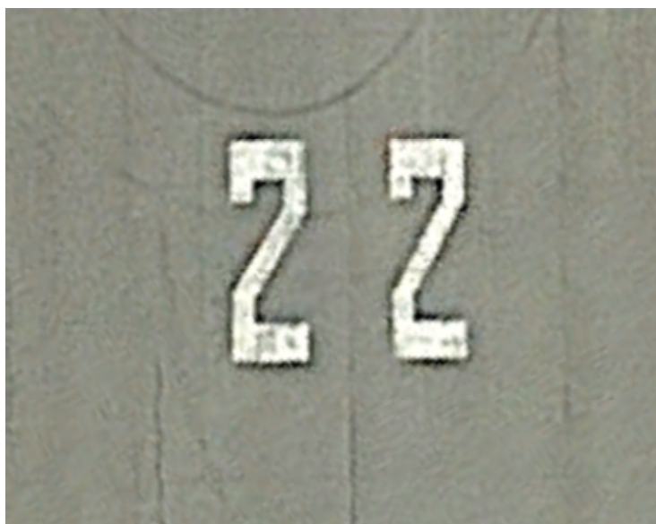
Figure 19 - Runway Designation Marking
