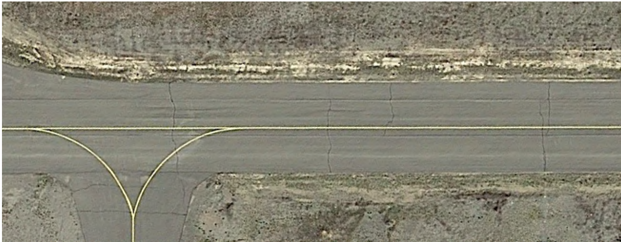
Figure 33 - Taxiway Centre Line
