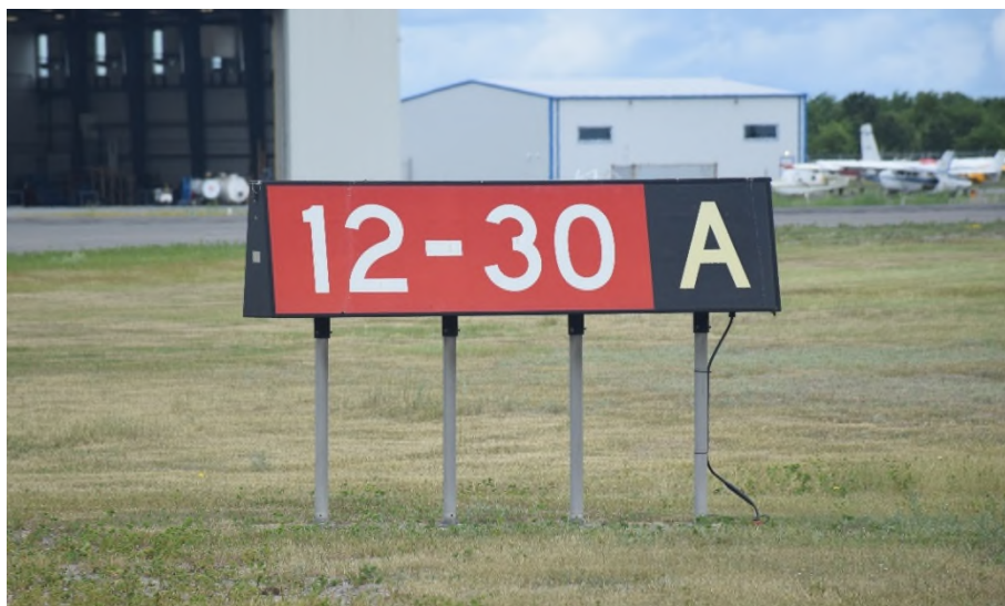
Figure 13 - Runway-Taxiway Intersection Mandatory Instruction and Location Sign
